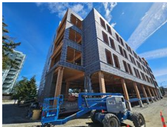
Wall panel installations looking east – May 2024
