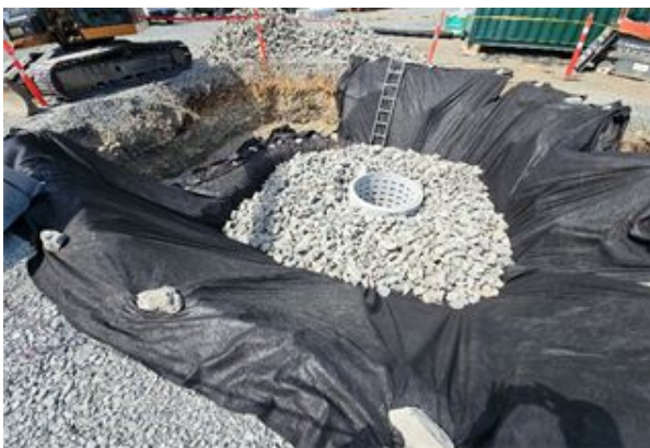
Installation of sump and drain rock – May 2024
