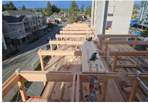
Site looking north (from level 3) – February 2024
