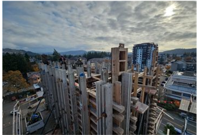
Site looking south (courtesy of Blackrete) – November 2023
