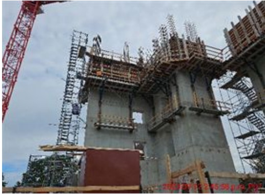
Elevator shaft level 4 to 5 – 12 September 2023
