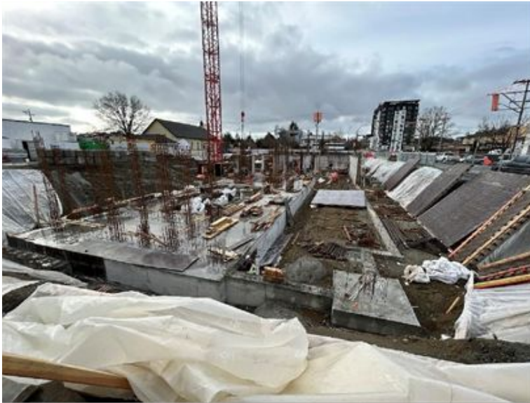
Phase I foundation and vertical structure, March 3, 2023
